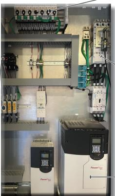
Motor circuit breakers, contactors, push buttons are on "Smartwire", a BUS system that allows for quick assembly, easy integration, and many diagnostic functions.
