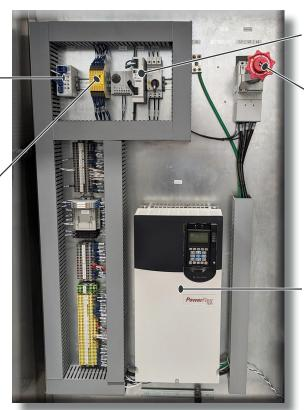
Power supply. Transforms AC line voltage and rectifies it into DC, typically 24V.
